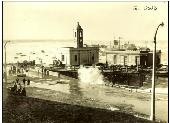
Sightseers at the Harbour as waves crash against the sea wall. The Lighthouse has already fallen and much of the Jetty walkway destroyed
