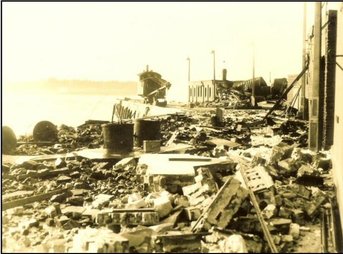
Wreckage on Margate Stone Pier after the storm. Part of the signage for Margate Surf Boat can be seen in the foreground on the right-hand side. Note the absence of the Lighthouse at the end of the Stone Pier
