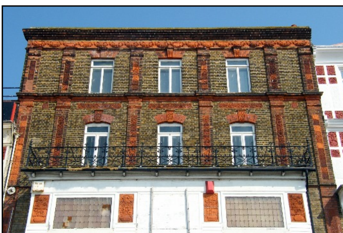
This photograph taken in April 2011 of the building on the right above shows some of the Aesthetic Movement terracotta panels which decorate the front of the property currently undergoing major works. It is believed that an additional storey is to be added to the property but that, importantly, the front elevation will remain unchanged
