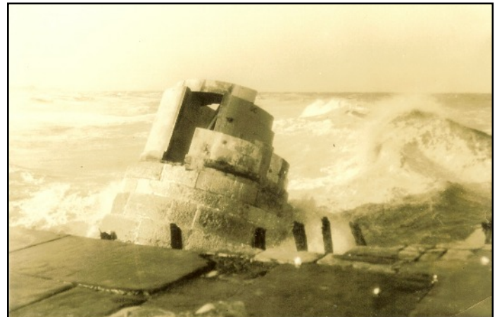
The old Lighthouse stood on wooden piles which gave way in the storm causing the Lighthouse to collapse into the sea. The base of the Lighthouse can be seen in this picture. The Lighthouse collapsed around 1.00pm on the day following the storm
