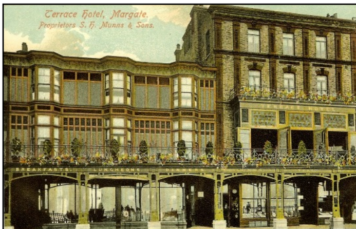
An Edwardian postcard of Munns Terrace Hotel and Restaurant on Marine Drive. It is the taller building that is being developed as the Sands Hotel. The building on the left was originally Phillpott's Hot & Cold Baths (see also 'Margate 1888' photo on page 11)
